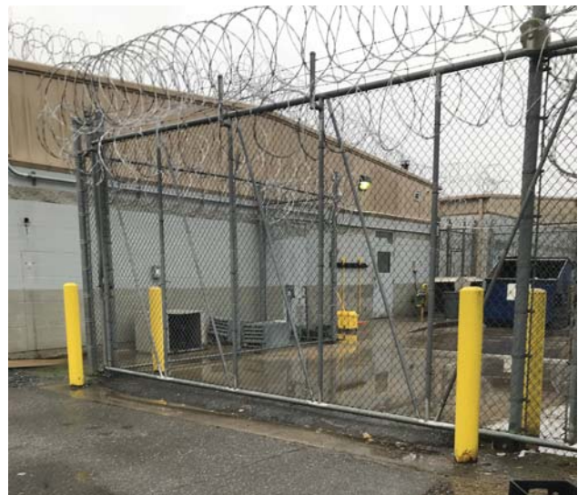
Entrance to Tallahatchie County Correctional Facility
